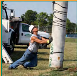
$14.9 M Infrastructure Investment
