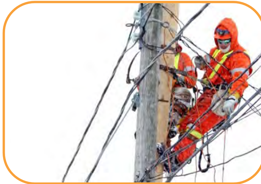
ENWIN crew members maintain lines in snowy weather.
